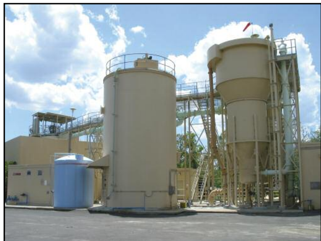
City of Temple Terrace Water Treatment Plant.
